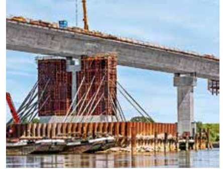
Vistula Bridge, Kwidzyn, Poland
