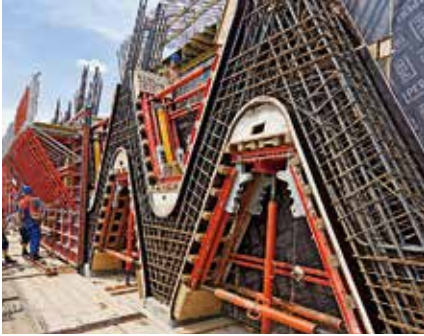
Prosta Tower, Warsaw, Poland
