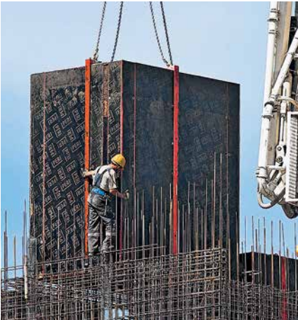
When pulling the Shaft Panels, a striking clearance of 3 cm is provided on each side, and the complete unit can be moved in one crane lift.
