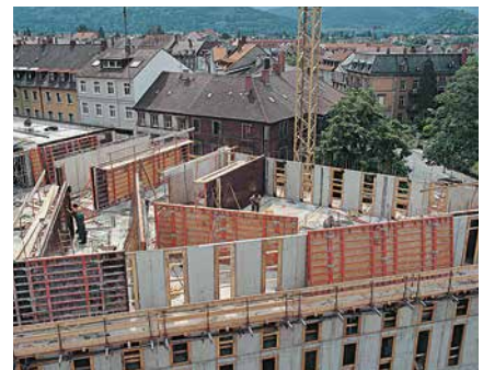
TRIO Structure can be combined with standard TRIO Panels. This is a great advantage as special surfaces are often required only on one side.
