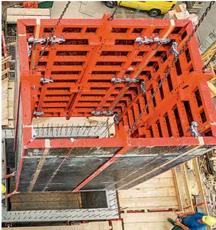
Rectangular shafts require adjustable crane slings due to the different lengths of the attachment points. This results in approximately the same tensile force on all four slings.
