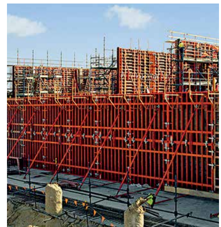
TRIO can be extended up to heights of 5.40 m in 30 cm increments. For larger heights, a compensation water is also used.
