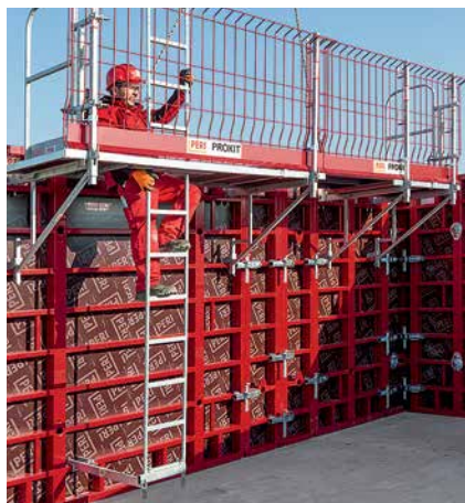
Standard assemblies of the MXK Bracket System are realized with 2.40 m, 1.20 m or 0.90 m widths.
