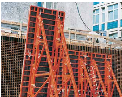
Friction-locked connections allow complete units to be moved.
