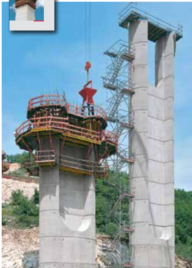
Motorway viaduct in France. Sophisticated pier geometry with an extraordinary concrete finish. Formed with VARIO GT 24 and SKS climbing brackets.
