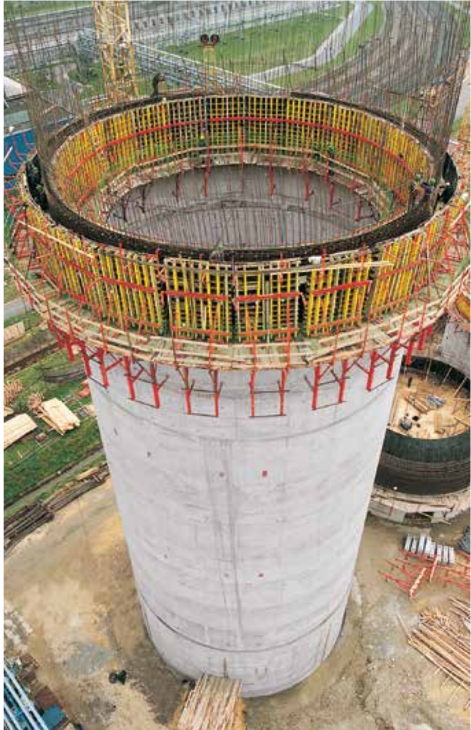
Silo, h = 72 m, Ø = 20 m for power station in Oppeln, Poland. Shuttered with circular VARIO girder formwork on KGF climbing scaffold.
