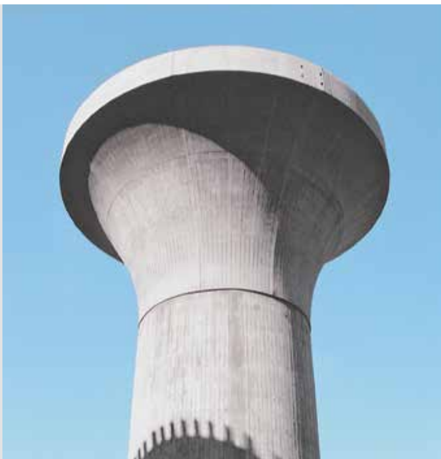
The BAB 4 motorway bridge over the Triebischbach valley was constructed with 49 m high circular piers featuring trumpet-shaped pier heads.
