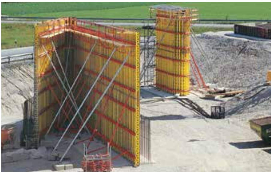
Abutment and bridge pier with VARIO GT 24. Crossing structure for the suburban railway line to the new Munich Airport.
