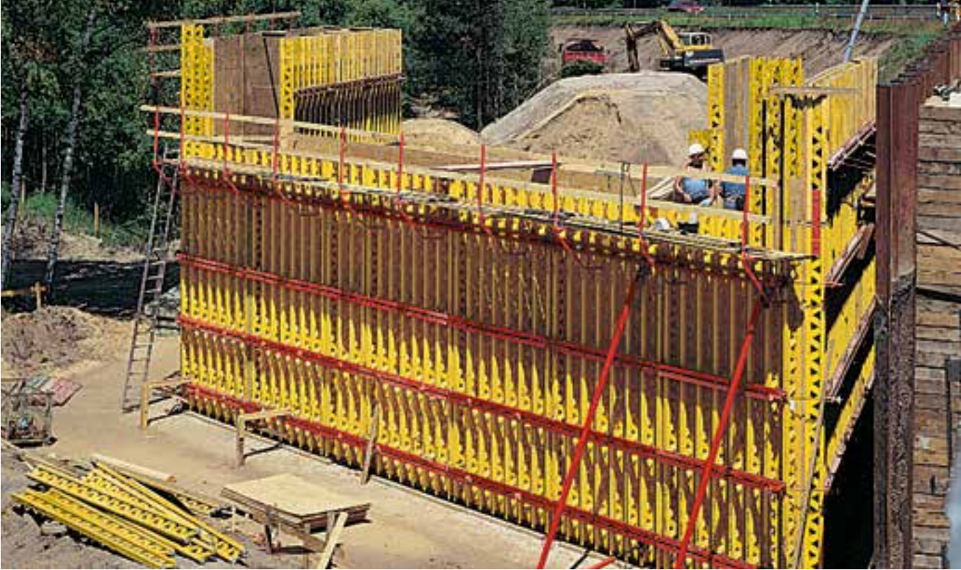
Bridge over the Danube, BAB 8 motorway near Leipheim.
