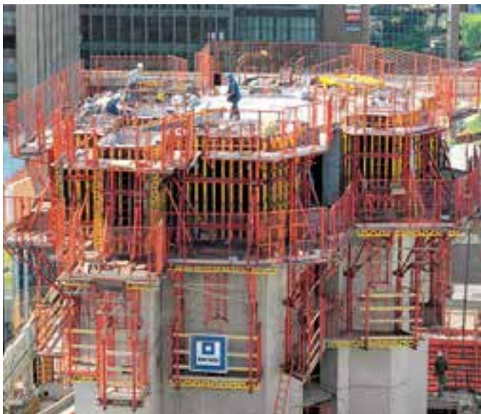
Multi-storey building in Paris with VARIO GT 24 and CB 240 climbing formwork systems.
