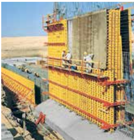
VARIO GT 24 being used to build a sewage treatment facility with tapered walls.
