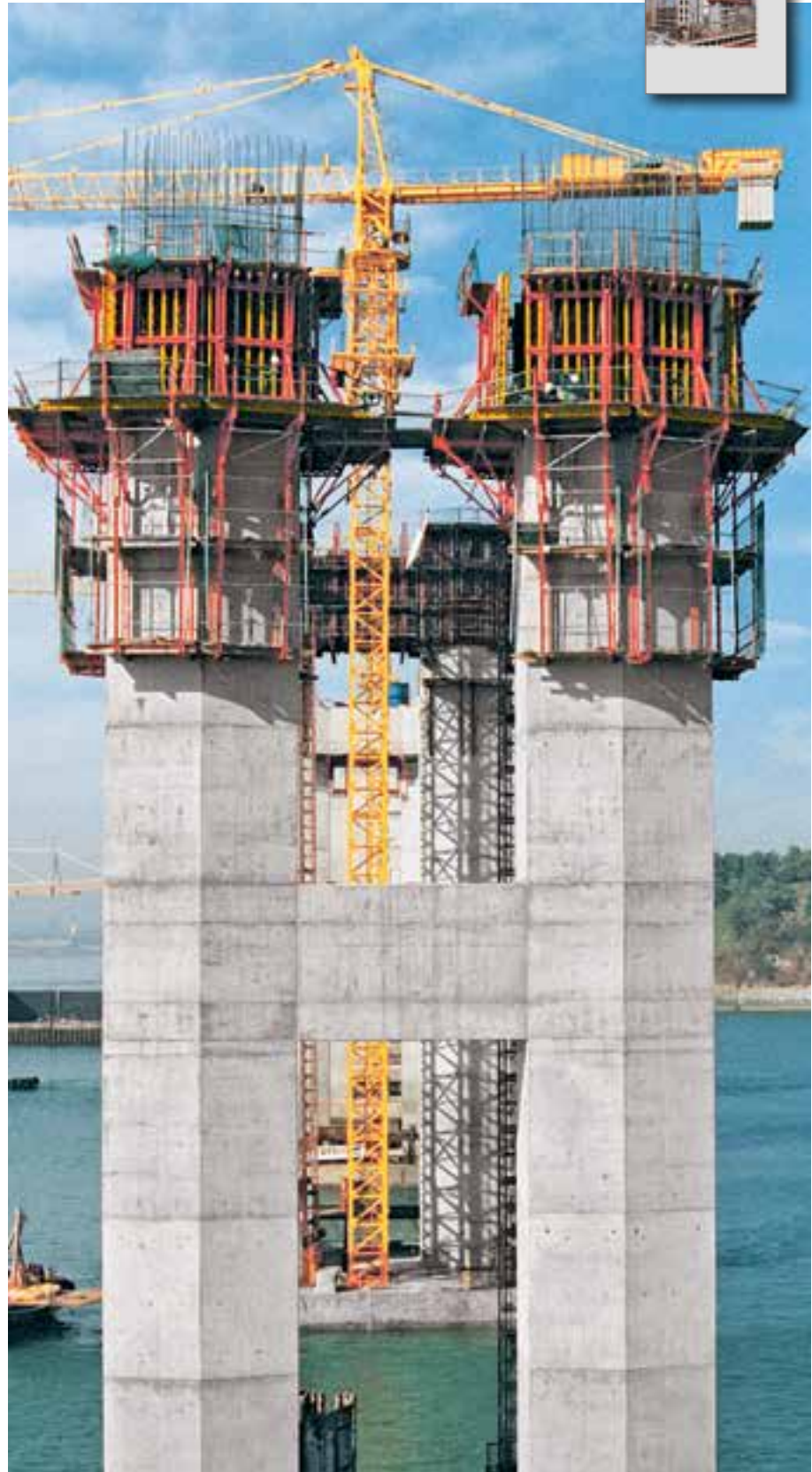
CB 240, the triangular bracket for problem-free working in front of and behind the formwork.
