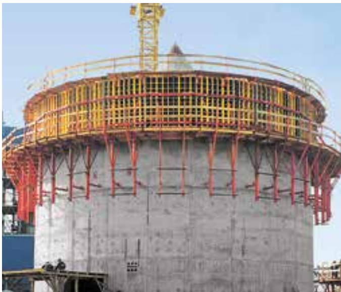
VARIO GT 24 being used to construct a circular tank. Timber wedges between girders and steel walers produce the circular shape.
