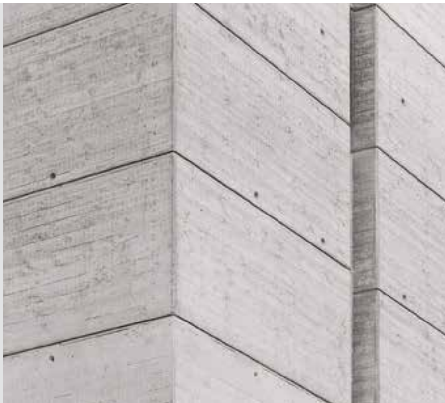
Exemplary fairfaced concrete with rough horizontal board finish.
