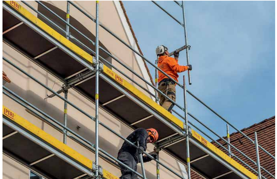
Fall protection without additional components thanks to the systematic assembly procedure with protection provided by the guardrail mounted in advance
