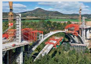
Bridge Formwork
