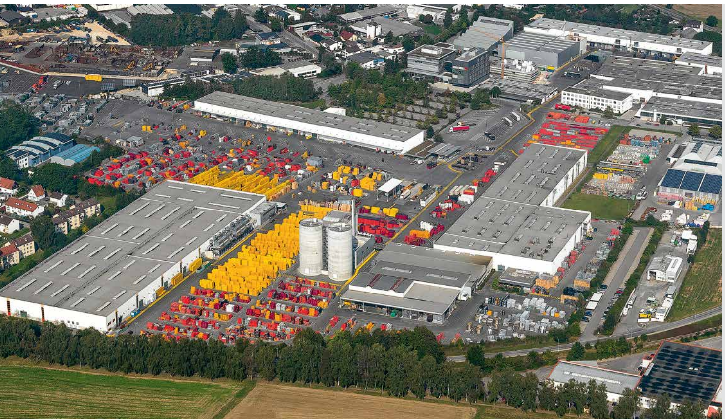
PERI in Weissenhorn: company headquarters, development and production.
