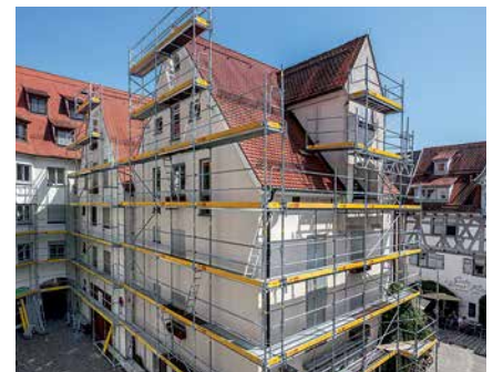
Assembly of the basic structure takes place virtually without any couplers, whilst the Easy quick anchoring system also reduces assembly times.
