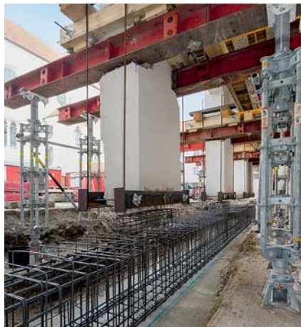
The 4-legged heavy-duty prop consisting of standard PERI UP system components can be used for transferring concentrated individual loads of up to 200 kN.
