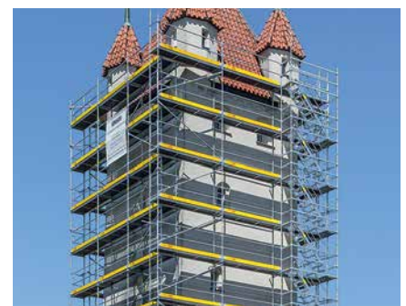
The Toeboard UPF is easily recognisable from afar due to the yellow signal colour.
