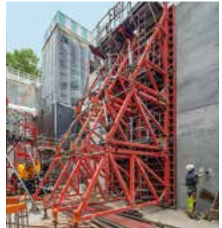
Through a corresponding assembly of scaffold tubes, the Brace Frame can be adapted to match the formwork regarding the width of influence.
