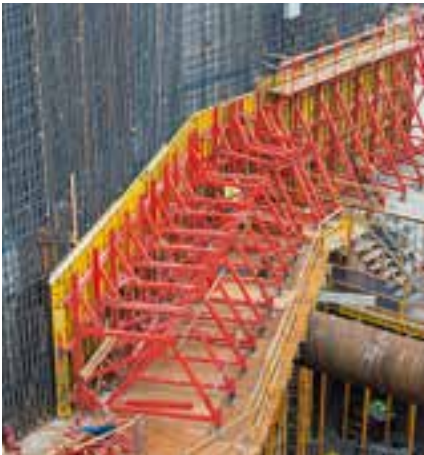
For lower concreting heights of 4.00 m, the frames of Brace Frames SB-A and SB-C can be combined.
