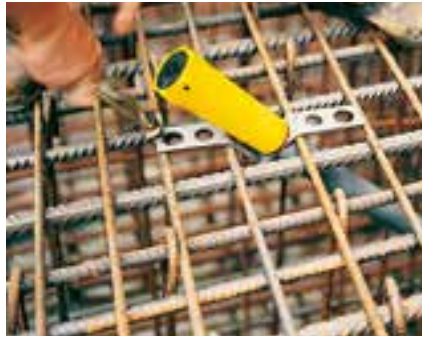
With the V-Tie Holder, as a lost part, an exact alignment of the Tension Anchor to 45° is possible.
