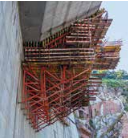
Brace Frames and system components taken from the VARIOKIT Engineering Construction Kit formed large-sized platforms up to 8.75 m wide.
