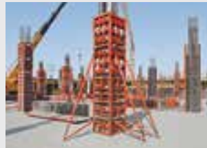
Column Formwork
