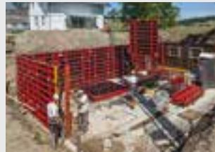
Wall Formwork
